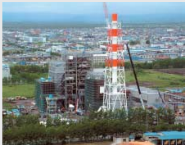
Constructing a wholesale electricity supply facility (Kushiro Mill)
