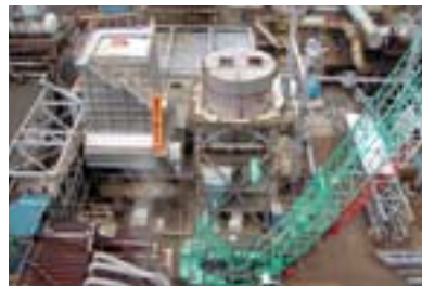
Biomass boiler under construction (Ishinomaki Mill of Nippon Paper Industries)
