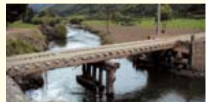
Wooden bridge constructed in collaboratively with local administrative agencies
